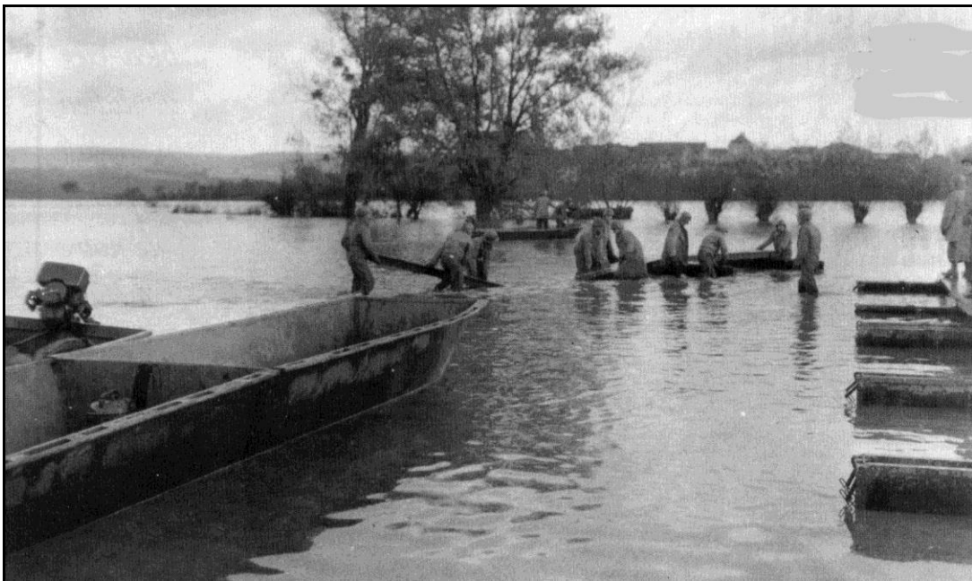
Construction of the pontoon bridge at Malling by American engineering troops. (Moselle River 44/Fund Rothenberger)
